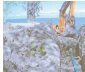
Excavating the toe
